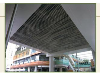
Design, supply and installation of external ceiling system at G/F for public rental housing development at Queen's Hill Site 1, Phase 1 & Portion of Phase 6 皇后山—號地盤(第一期及第六期部分地盤)公共房屋發展項 目一設計、供應及安裝地面層之室外天花系統
